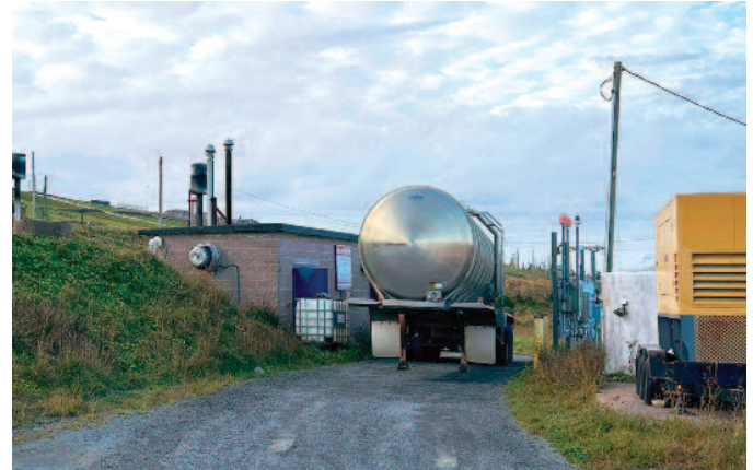
The brick building at the Otter Lake landfill contain blowers that suction the methane and the sulfur compounds found in landfill gas from the waste burial cells through a pipe network. The large tank fills with condensate; flares from the larger pipes burn the gas, and the smaller pipes relieve pressure. Photo: Jason Timms
